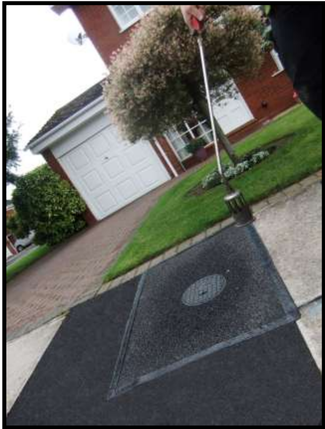
Heron Close, Worcester Water meter installed using Ultracrete's Reinstatement System
